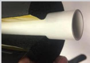
Wrap around the pipe, peel away yellow cover and seal together. Use the adhesive flap to secure.
